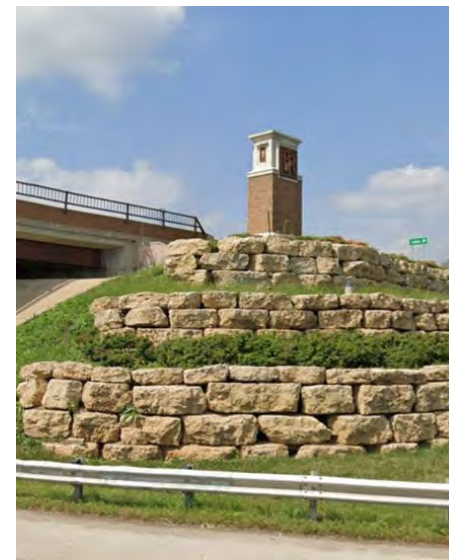
I-55 at Bolingbrook
